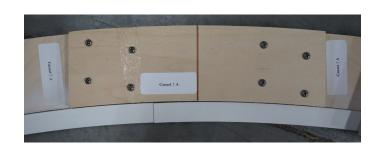
Once joints are secured, assembly is turned right side up and section of perimeter angle which laps over joint is secured with #8 x 3/4" truss head provided.
