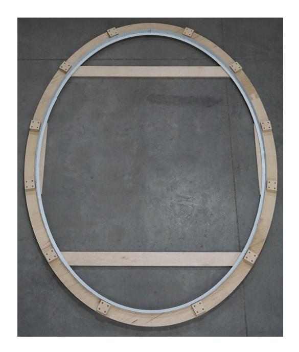
A Perimeter Assembly: the four sections have been locked together at the joints, secured with gusset plates and the assembly has been turned over in preparation for installation.
